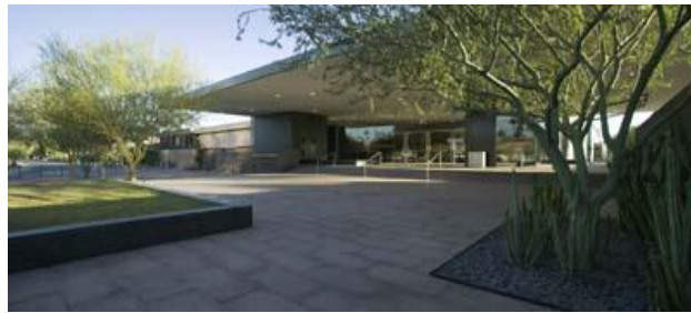
Figure 2. Exterior view of the Phoenix Art Museum, Phoenix, Arizona.
